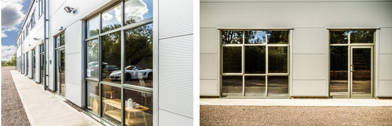
Smarts Shopline is a **non-thermally** broken system designed for all ground floor treatments and high traffic doors
