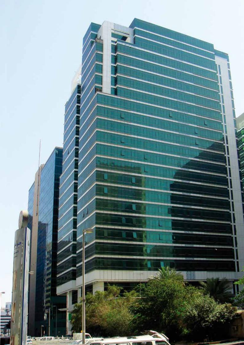
Elegance 52 SG is a structurally glazed curtain wall system using the basic substructure of Elegance 52 and offering a solution for combinations of fixed or opening panels in both straight or facetted applications. The structurally glazed curtain wall offers a minimal sightline without having a visual difference between fixed and opening panels.
